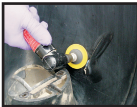
Prepare the damaged area
