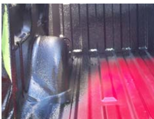
Truck bed in progress.....
